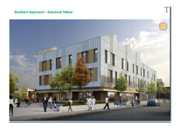
The dimensions of the building are a foot print of 21m (W) by 45m (L) 8.3 with an overall height of 16.2m to the saw tooth apex reducing to 13.2m to the flat roof. The concept of the building is a grid shape of rooms which would be 7m by 7.5 metres (see ground floor plan arrangement below).
